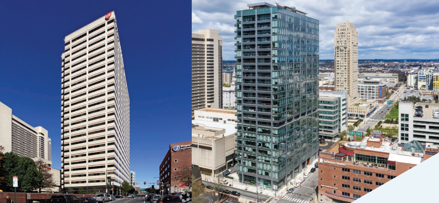
The office building to the left was reclad with energy-efficient glass and aluminum framing. Courtesy CoStar. ■
