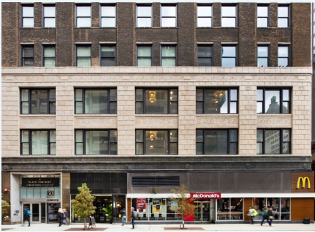
The conversion of the building preserved its historic façade. Courtesy SPACE Architects + Planners. ■
