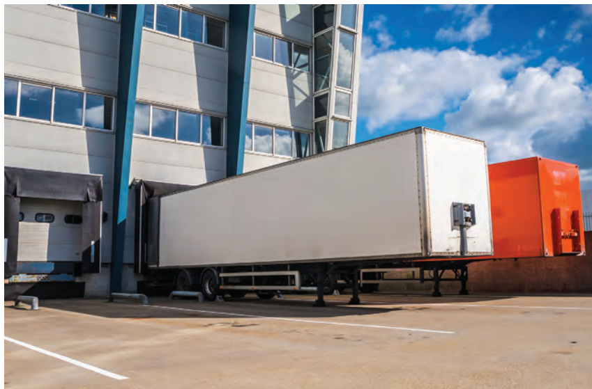
The number of loading docks is one of many factors a tax appraiser might consider when calculating property tax for an industrial facility.
