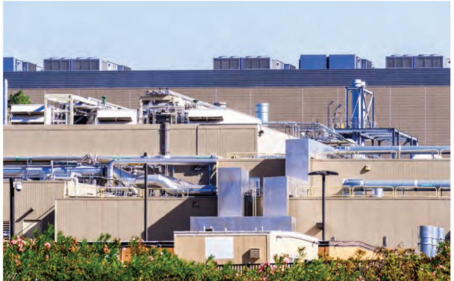
Data centers face unique challenges around power demand because of the huge amount of cooling that is required to keep the servers operating.
