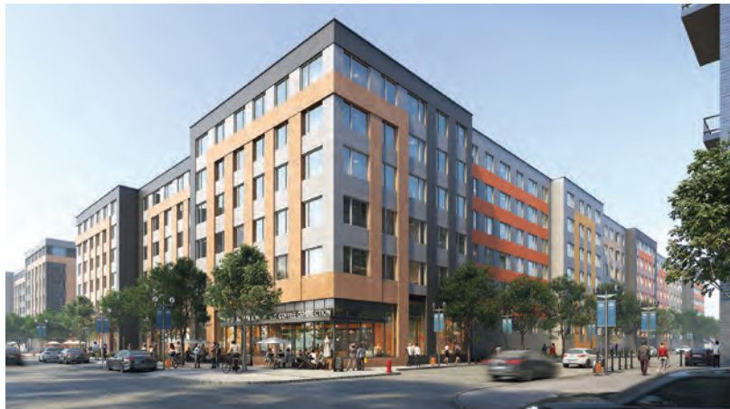
When it's finished in May 2025, Greystar's The Maxwell will consist of 355 market-rate apartments, 29 affordable-housing units, a parking garage with 460 spaces, and roughly 5,300 square feet of retail space on the ground floor.
