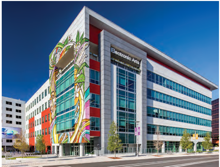
Electronic Arts (EA) recently moved into a newly built 180,000-square-foot building in downtown Orlando's Creative Village, a 68-acre mixed-use, transit-oriented development.
