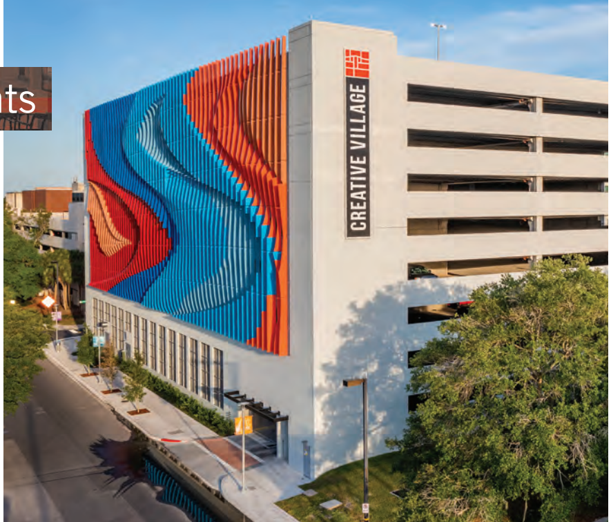
The parking garage for EA Sports' new headquarters in Orlando features an undulating façade that hides the facility and evokes the world of virtual reality.
