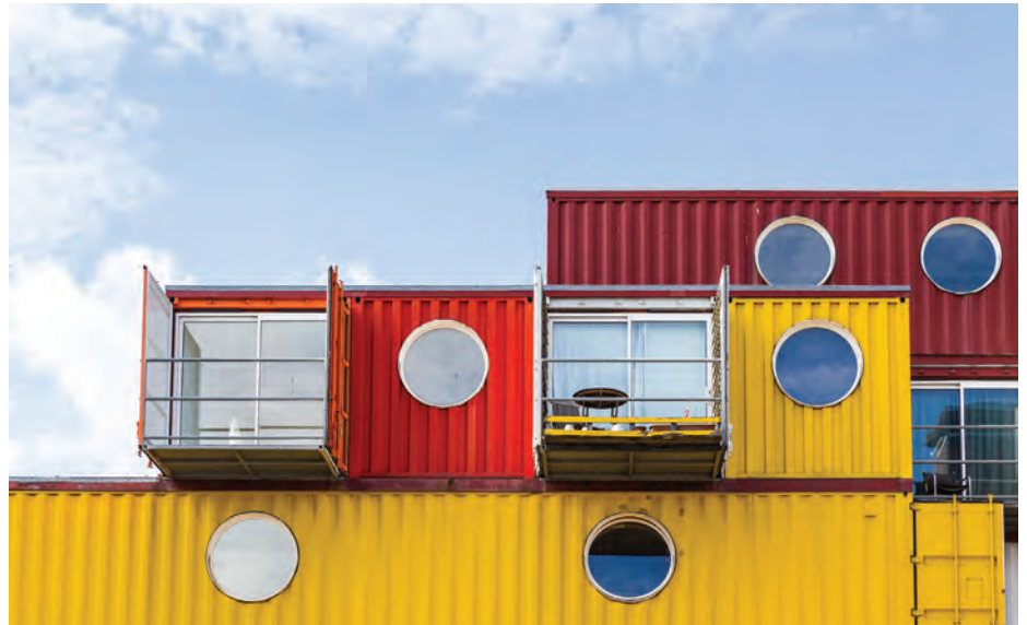
Trinity Buoy Wharf is an arts and cultural center in London that includes several workspaces and offices built out of shipping containers.
