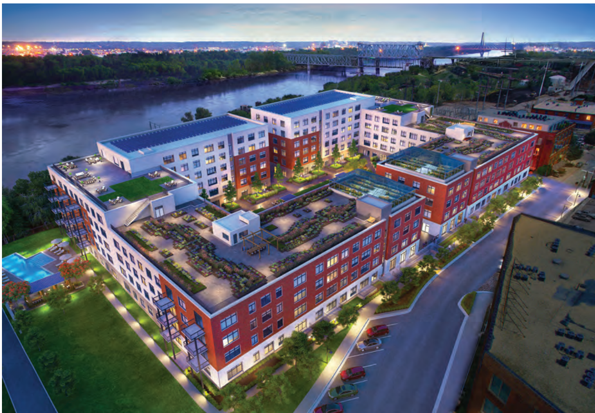
At 276 units, Second + Delaware, in Kansas City, Missouri, claimed to be the largest passive-building multifamily project in the world when it opened in 2020.
