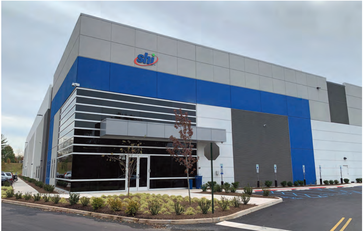
SHI International, a provider of information technology (IT) products and solutions, has a 396,750-square-foot building in the Rockefeller Group Logistics Center. The original design was altered to accommodate the company's IT configuration work. The finished facility has greater HVAC capacity, a depressed slab, increased electrical service and solar panels on the roof.
