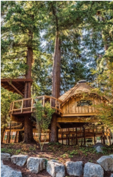
Outdoor Meeting Space One on Microsoft's Puget Sound headquarters campus features a 900-square-foot circular conference room and deck, accessed via a 250-foot ADA-compliant ramp.
