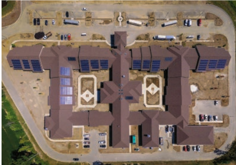
Social Row Transitional Care Center, shown here under construction in August 2017, features protected courtyards as well as rooftop solar panels, which were financed in part through PACE financing.
