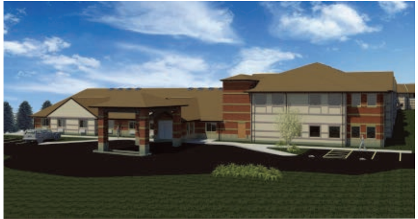
Challenging site conditions required a three-story addition to the Forest Hills Care Center. This entrance will provide access to the assisted living and skilled nursing units. A separate entrance on a lower level will provide access to a new physical therapy gym, enabling Forest Hills to provide outpatient PT services without disturbing residents.
