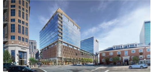
includes two Class A office towers with 20,000 square feet of street-level retail space. The steel-framed glass structures rest atop a post-tensioned concrete-framed seven-level parking structure. At the top level of the parking structure, a 45,000-square-foot open-air garden terrace will serve as a signature amenity and be available for public events. The project is expected to be completed in the summer of 2022.
