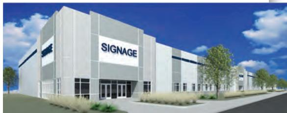
feature clear heights of 28 feet and eco-friendly, insulated wall panels. The site is located minutes away from I-35, K-10 and I-435 highways.
