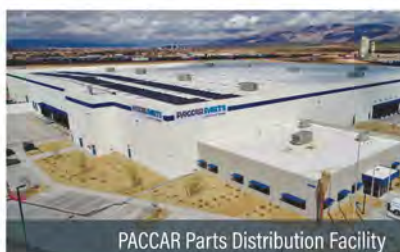
PACCAR Parts Distribution Facility
