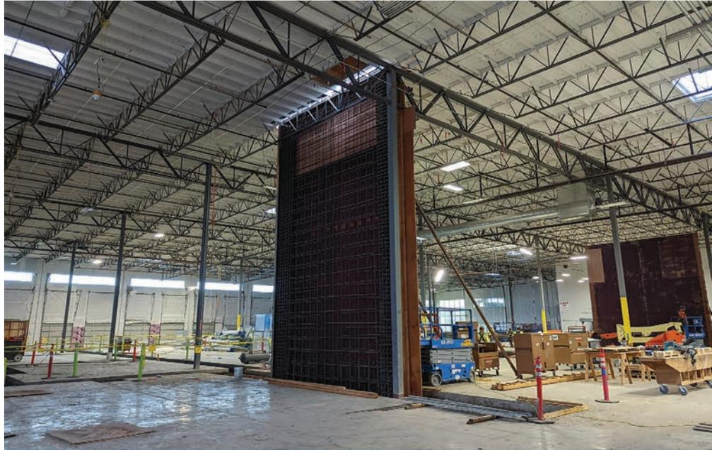
One of the nine concrete shear walls, measuring approximately 30 feet tall, installed inside of the existing tilt-up warehouse.
