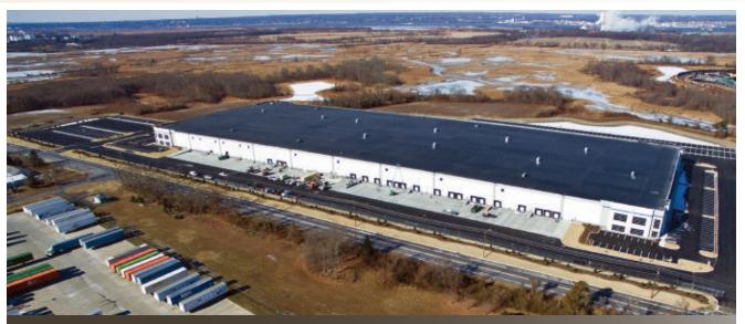
The building's primary tenant, a distributor of motor oils and industrial lubricants, had specialized environmental and safety requirements, including interior and exterior systems to prevent spills from getting into the sanitary sewer system as well as ESFR fire protection with sprinkler heads installed near product storage areas.
