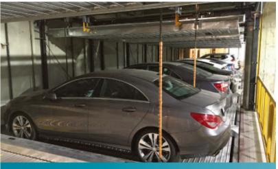
A three-level semi-automated parking system at the Idora Apartments in Oakland, California, enables the facility to accommodate 42 cars on a site area that could accommodate only 15 standard surface parking spaces.
