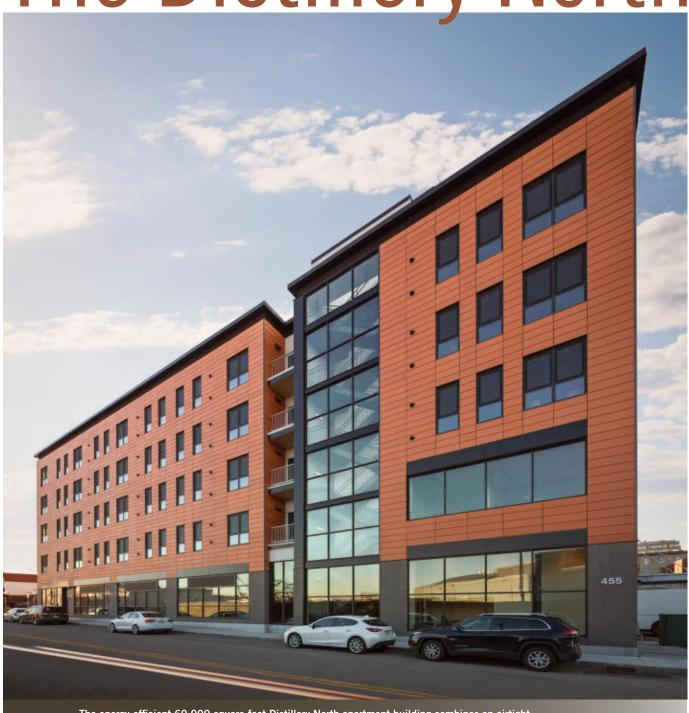
The energy-efficient 60,000-square-foot Distillery North apartment building combines an airtight building envelope with intelligent ventilation and careful attention to solar gain.
