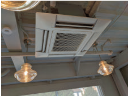
Incorporating recessed cassette units rather than ducts enabled designers to maximize the building's ceiling heights
