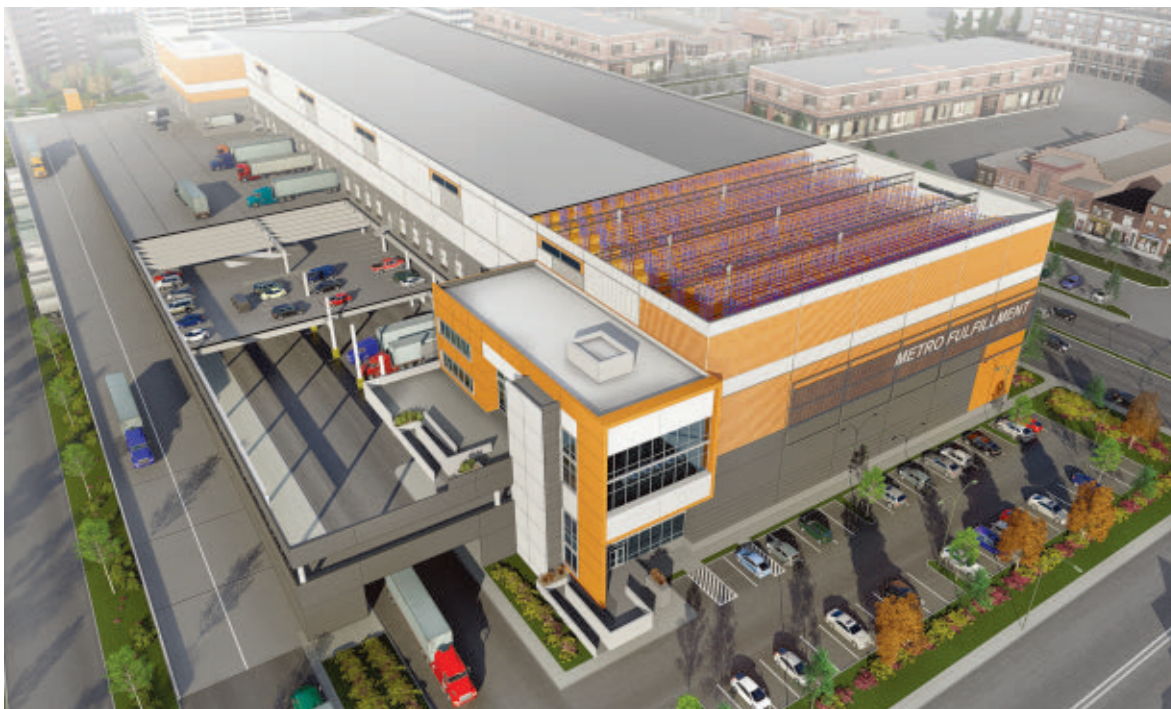
E-commerce capabilities and auto parking integrate into a two-level fully functional truck court (at left in rendering above). A parking deck inserted between the upper and lower truck levels creates a functional queuing area for last-mile delivery vehicles while also providing a large number of parking spaces.
